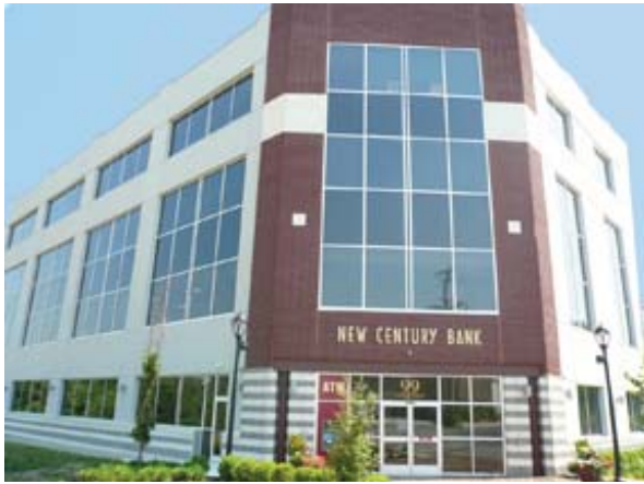
New Century Bank Mini-Branch Entrance
