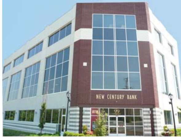
Exterior view of Mini Branch
